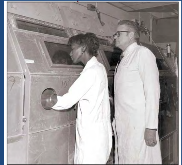
Neptunium billet line glovebox worker (1978) SRS at Fifty – Reactor On (2002) (SRDB 24750)
