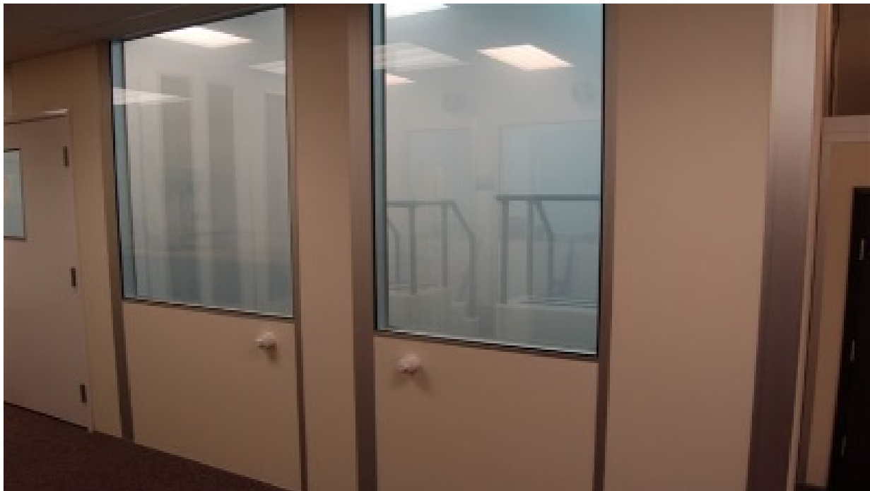
Figure 6: Charged Test Chamber
