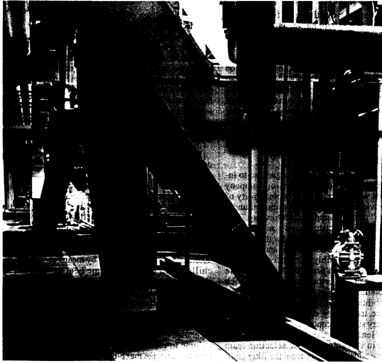
Filter with inclined conveyORIZED chute extension discharges chips into an in-floor cross conveyor. Chips are transferred out of the galleries to large dump trailers for transport to a salvage operation
